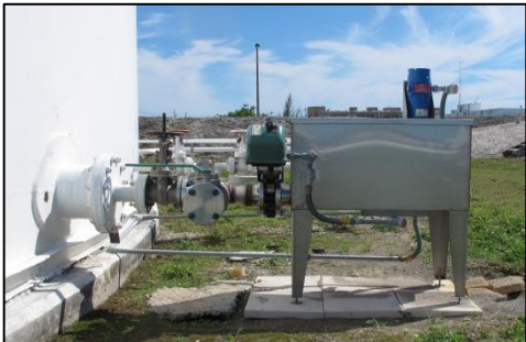
Tank Farm / Storage Facility
