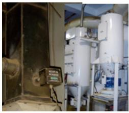
Cyclones on Drying Plant protected by fully insulated sensors
