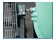
Pro-Scatter and Electrodynamic Main Stack Sensors
