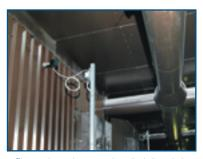
Electrodynamic sensor installed directly in Baghouse compartment wall
