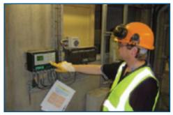
PCME systems allow the safe examination of the filter either at the control unit or remotely via a PC
