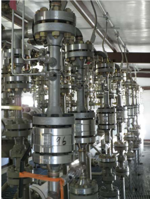
Figure 2: Installed V-Cone Flowmeters
