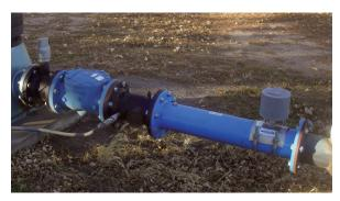
Figure 4: Mc Propeller Flow Meter With Integral Flow Straightener Installed At A Pump Station
