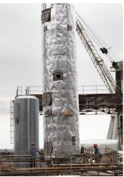
The ECO-EGC<sup>TM</sup> OPEN LOOP system, uses only seawater to neutralize the SO2 contained in the exhaust gas.
